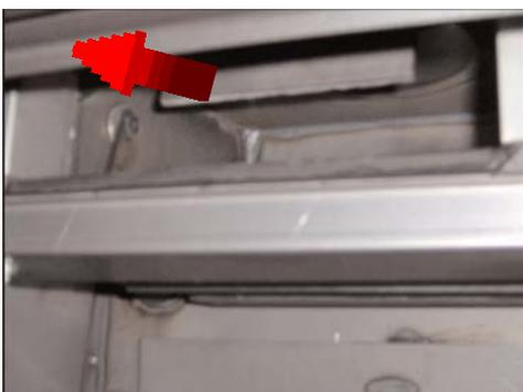
Now that the combustor has been removed you'll be able to see one stainless bypass retainer on each side. These can remain in place and do not need to be removed. Using the same screwdriver or pocket knife, scrape any old gasket from the surface areas of the dome. If you clean your existing combustor you'll need to order replacement combustor gasket. If you purchase a new combustor a new gasket will be applied to the combustor.
