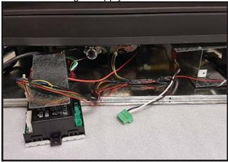
Plug green blower connector into the IFC control box.
