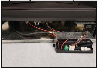
Slide blower through left-hand side to the back of appliance. Slide wires beneath the valve. Ensure wires do not get pinched or hooked anywhere.
