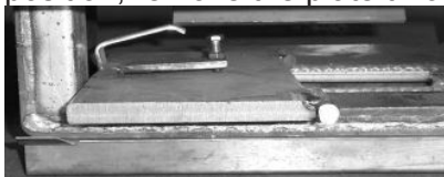
BYPASS DOOR REMOVAL THROUGH COMBUSTOR OPENING
