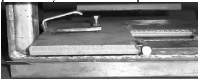
BYPASS DOOR REMOVAL THROUGH COMBUSTOR OPENING
