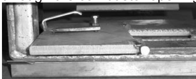
BYPASS DOOR REMOVAL THROUGH COMBUSTOR OPENING
