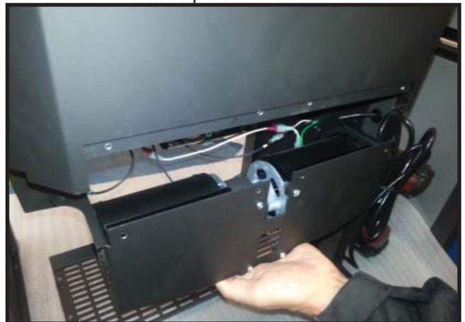
Ensure the side tabs are between the support panel and the firebox bottom panel.
