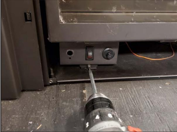
9. Pull the control panel out in front of unit. Remove the knob, nut, and washer from the rheostat.
