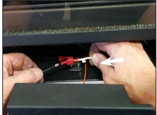
13. Fasten the ground from the power cord to the front firebox leg.
