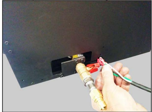
6. Slide the loomex bushing into the case hole.
