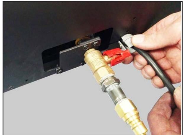
7. Rotate the loomex bushing so slots are offset.
