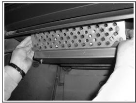
8. When correctly installed, the flame shield will rest on the two tabs located on the dome guard and will lean slightly forward. Now that the combustor and flame shield have been properly reinstalled, the appliance can be relit.
