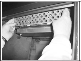
2. Once the flame shield is removed, you will have access to the combustor. The combustor can be made of different materials such as cordierite, mulite, or stainless steel. They are all the same with regard to removal and caution should be taken so as to not drop or damage the combustor. If your combustor has never been cleaned according the manufacturers directions, you may wish to clean the combustor before replacing it with a new combustor (please refer to the "COMBUSTOR CLEANING" section).
