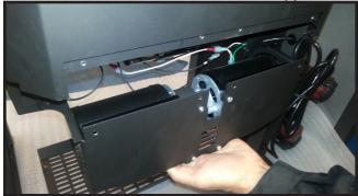
3. Secure the fan by fastening x6 screws to the appliance (note: x2 screws fasten into the firebox bottom).
