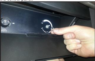
Slide the control knob onto the rheostat post.
