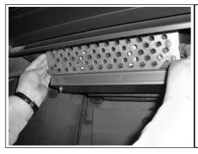
1. The appliance must be cool to touch, having gone at least 12 hours without being burned. A combustor can reach 1400F and hold temperatures for several hours, even after the fire is out. After waiting 12 hours, begin by removing the flame shield by simply lifting the shield off the two tabs at either lower corner. Pay particular attention to orientation of the flame shield in order to reinstall in the correct position.
